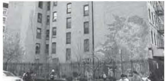
Condition of The Mural in August 2009 (Photo by Tomie Arai)
